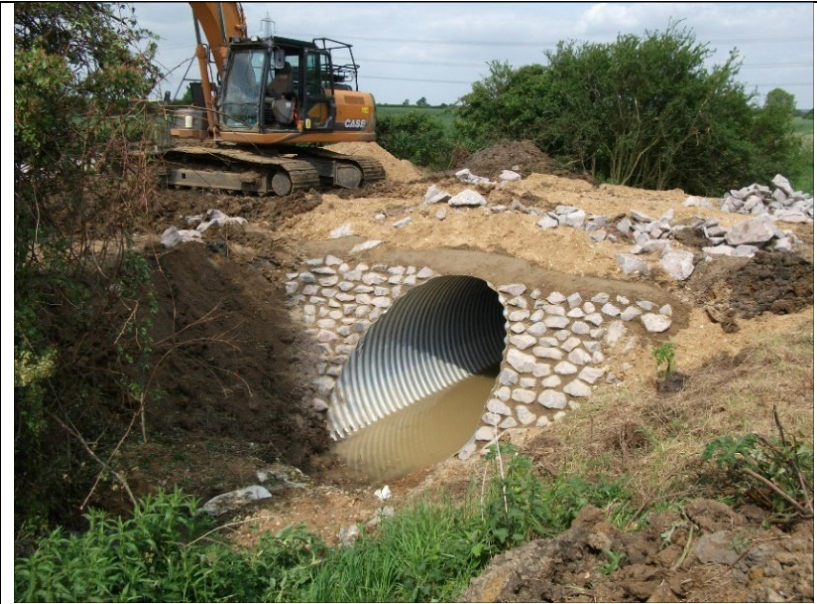
A culvert being installed
