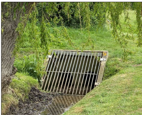
The culvert weedscreen
