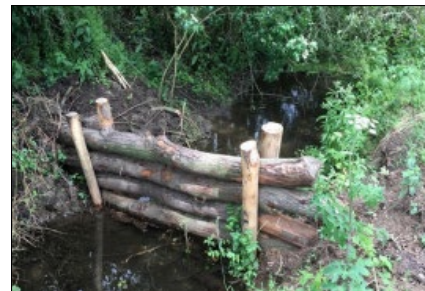
A woody debris dam.
